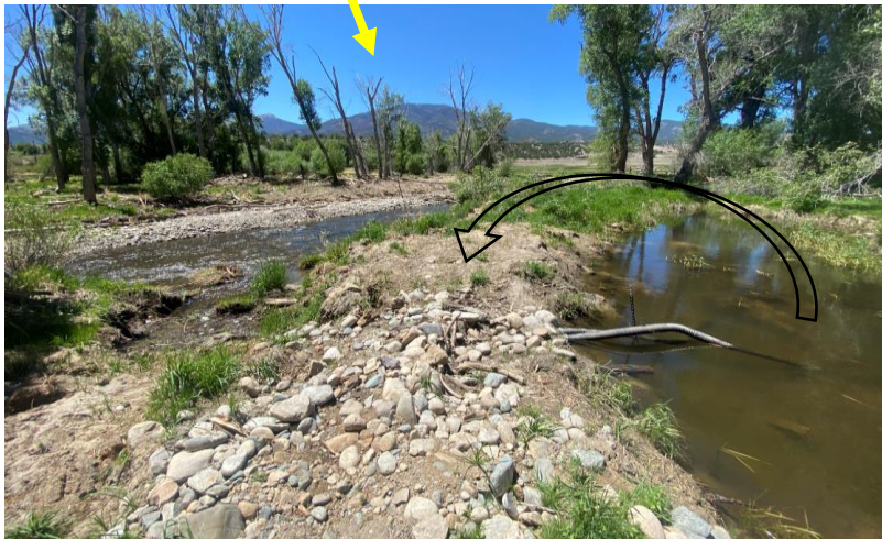
↑ A levee built to create a dam for an off-channel pond.
